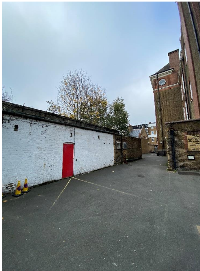
Image 4: View of outbuildings to be demolished
